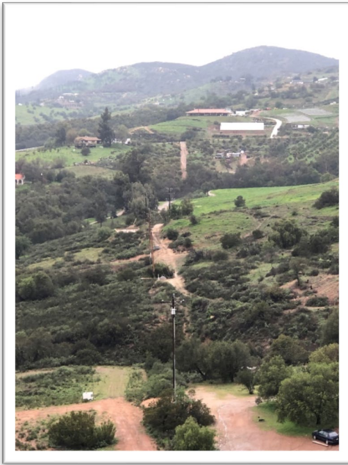
Valley Center Municipal Water District Pipelines Replacement Program, San Diego County
